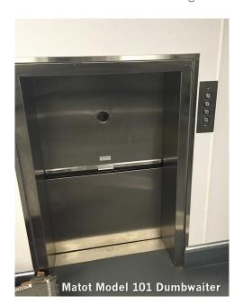
The Matot Model 101 Ambassador Drum Dumbwaiter is 36 inches by 36 inches and has a total load capacity of 500 pounds. With a total travel time of less than nineteen seconds between floors, the Matot dumbwaiter increases the efficiency of the Deer Path Inn wait staff by allowing them to roll heavy carts of food to the dumbwaiter and shuttle them between floors.
