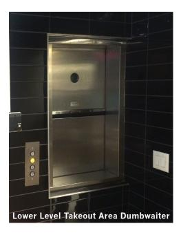
Matot was proud to custom design a dumbwaiter to meet these challenges. The Matot Model 110 dumbwaiter has a 200 lb capacity and a 24 inch by 24 inch by 36 inch cab, giving it the ability to handle large heavy trays of food. With a 17 second travel time between floors, the Matot dumbwaiter quickly transports food orders from the kitchen to the takeout area below.
