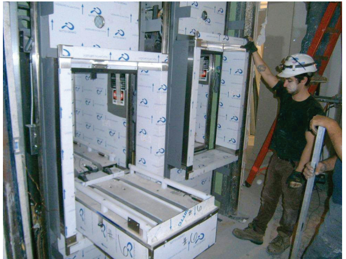
A Matot dumbwaiter with the automatic tote conveyor next to a standard dumbwaiter during the final stages of installation
