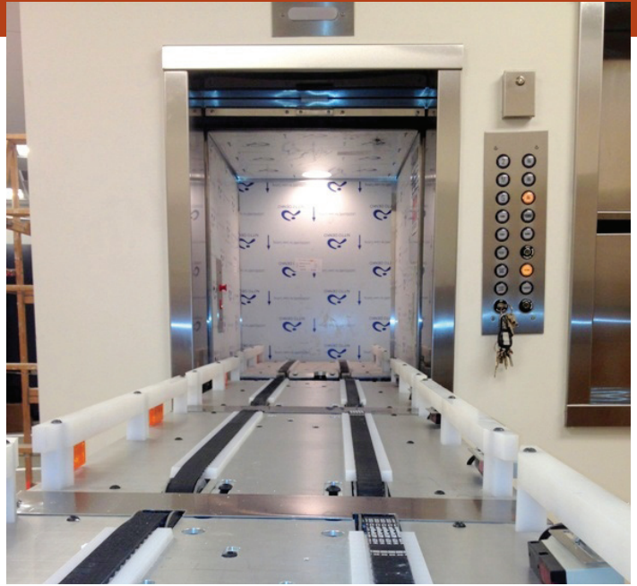
Matot dumbwaiter with an automatic tote conveyor installed in Macy's flagship store in New York City.
