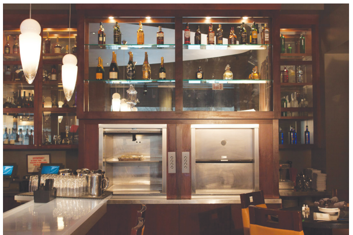
Matot counter-loading stainless-steel dumbwaiters side by side at Devon Seafood Grill in Chicago
